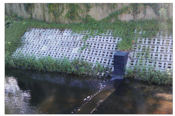
Eight (8) Weeks After ACBM install. Planted vegetation taking over through Open Cell ACBs
