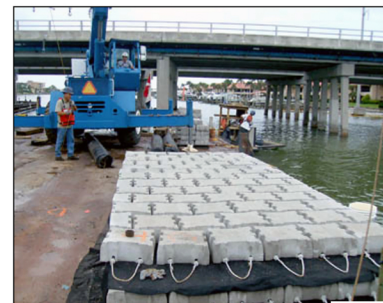
Preparing ACBMs for Install
