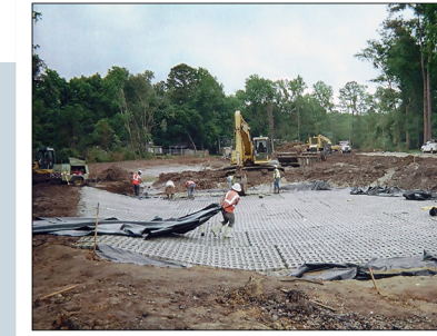
Open Cell ACBMs during installation
