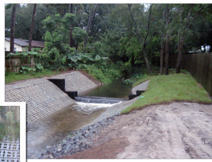
Two (2) Days After ACBM install
