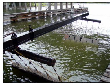
Spreader bar lowering ACBMs into underwater position.
