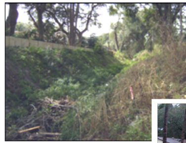
Before ACBM install
