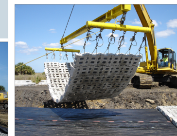
ACBMs during install
