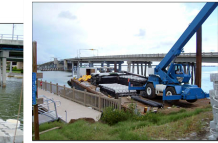
Barge Loaded for ACBM install
