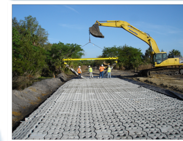
ACBMs during install
